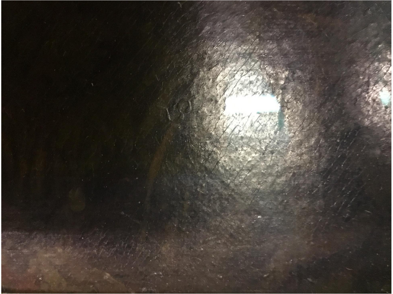
5. Minor Cracking Lower Right Corner D / Cracks / 11 Aug 2017 / Detail of 1. Overview Front
