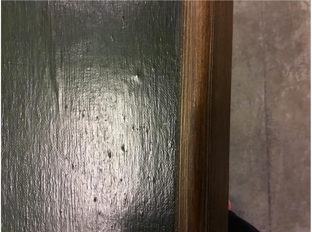
2. Small Chip Top Centre A / Flaking / 14 Aug 2017 / Detail of 1. Overview Front
