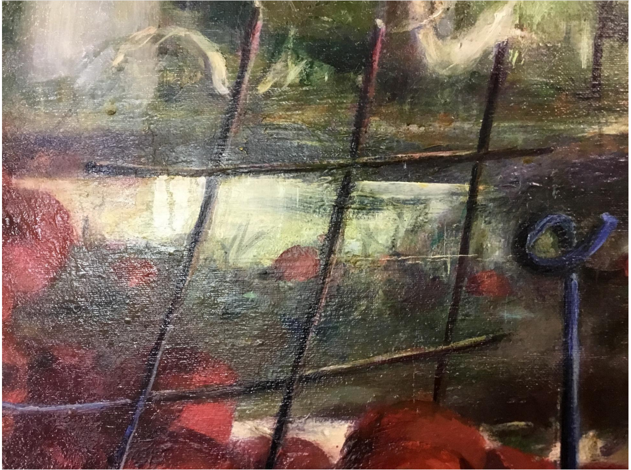
3. Cracking Lower Left Centre B / Cracks / 14 Aug 2017 / Detail of 1. Overview Front Left
