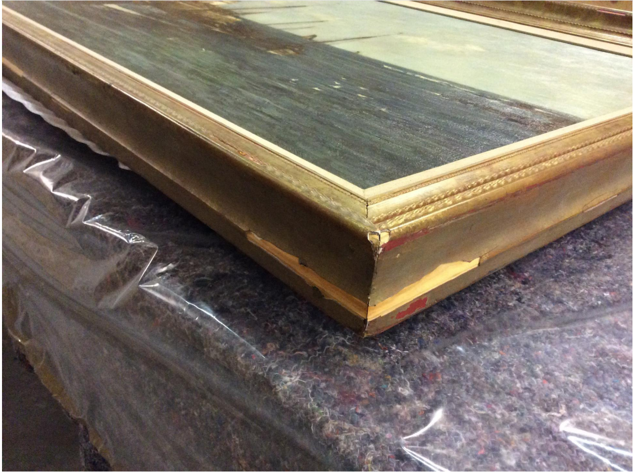
11. Chip To Frame Lower Right Corner H / Knock, corner / 11 Aug 2017 / Detail of 1. Overview Front
