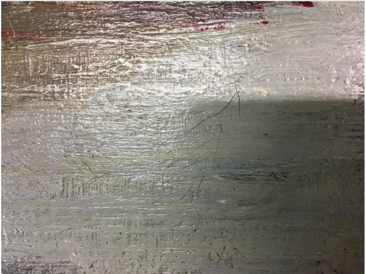
2. Cracking Lower Left A / Cracks / 11 Aug 2017 / Detail of 1. Overview Front
